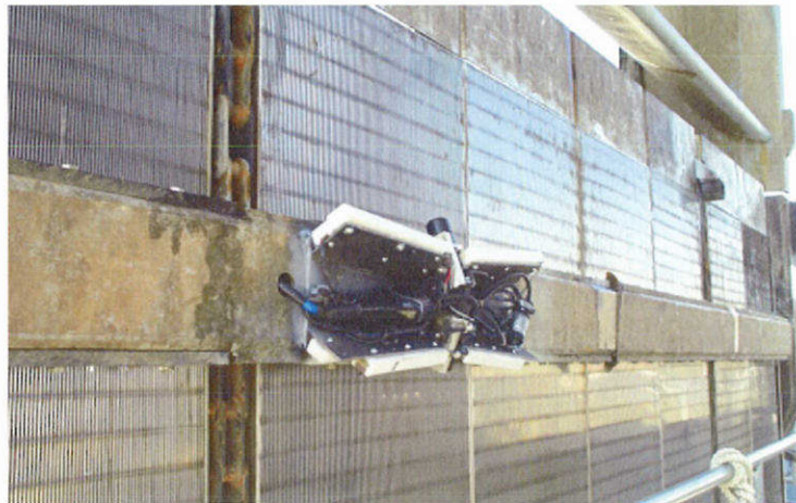
Figure 8. Underwater Cameras and Infrared Lighting Mounted on Brush Bar
